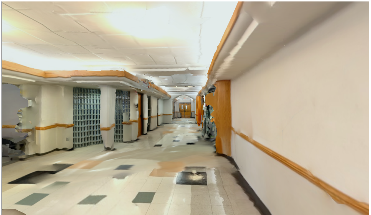
Figure 7: East-facing screenshot of Albertson Hall
